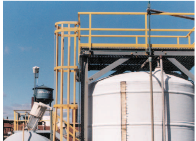
This fiberglass ladder and ladder cage provide worker access to a maintenance platform at a Ciba Geigy plant in the northeastern United States.
