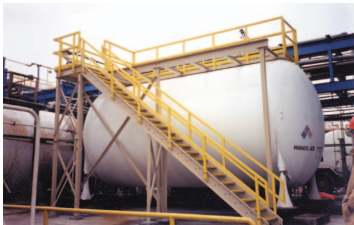
SAFRAIL™ system in a chemical plant.
