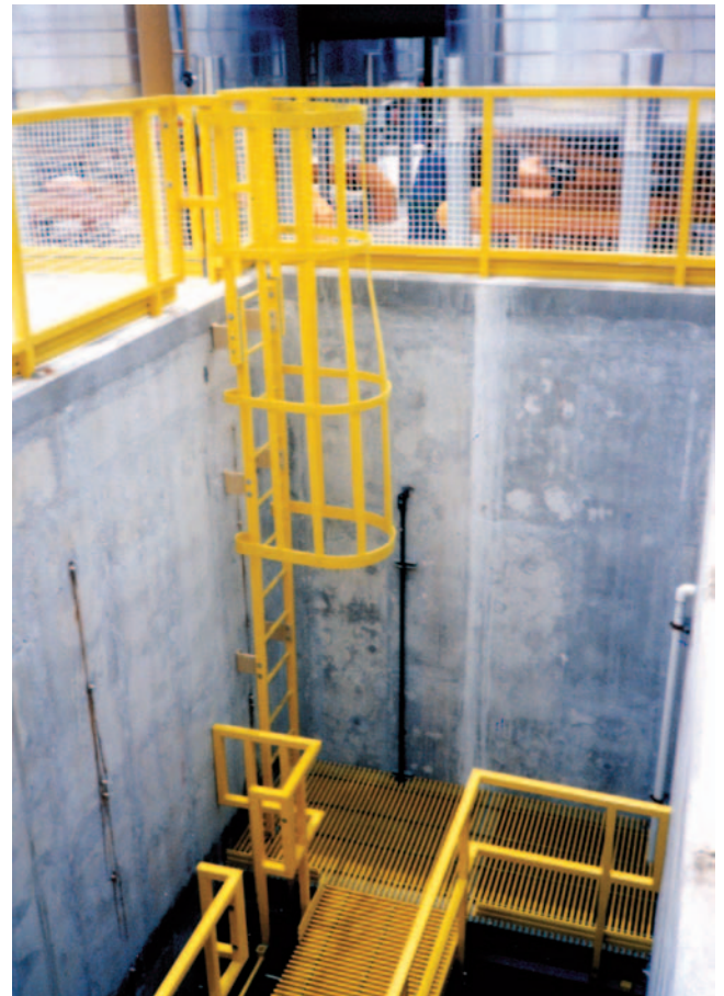
Fiberglass access ladders are used throughout the service areas of Sea World, Orlando, FL to resist saltwater corrosion and reduce maintenance
